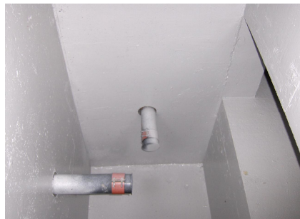
Finished concrete part
