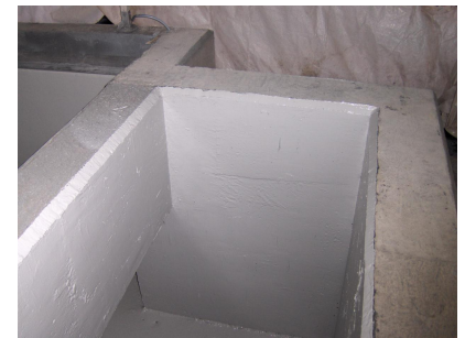
Finished concrete part
