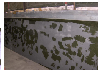
Wall touch up of cellar
