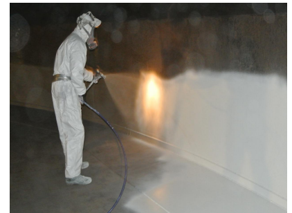
Single layer application of tank floor and wall
