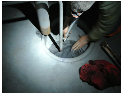
Vacuum cleaning of the tank floor
