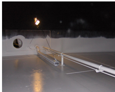
Average DFT 700µm, no pinholes found
